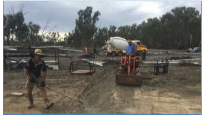
Garage under construction (Geoff Gowty in charge!)
