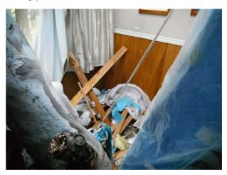
This limb broke off the tree and fell hitting the ground leaves first. The compression of the springy braches caused the limb to become airborne, travel some metres through the air and land butt first through the roof of the cabin, through the bed in the cabin and through the floor. Luckily the cabin was unoccupied at the time.
